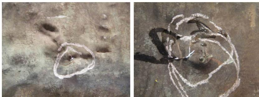
**Figure 7.** Details of roof panels – cracks and penetrations (lower side of copper sheets).
