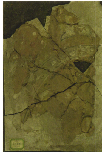
图9 支撑体断裂致使壁画开裂、变形 Fig. 9 The cracks and distortion of the wall painting caused by the break of support
